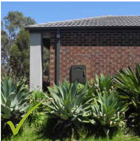
Example of meter box on side of house screened by planting and painted to match the downpipe and house.
