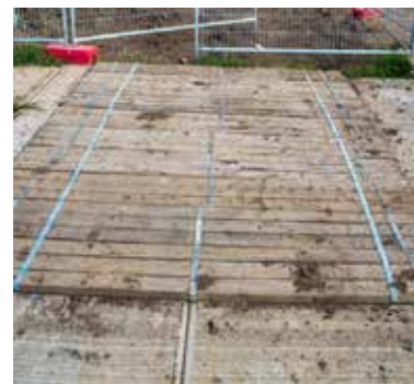
Example of wooden driveway crossover protection during construction of house.
