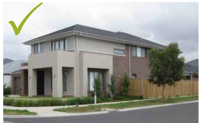
Examples of double storey houses with well-articulated facades facing onto secondary street, using the same materials, finishes, colours and facade articulation.
