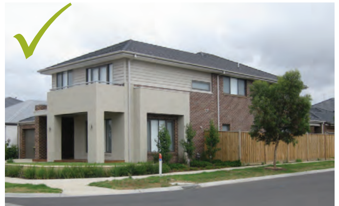
Examples of double storey houses with well-articulated facades facing onto secondary street, using the same materials, finishes, colours and facade articulation.
