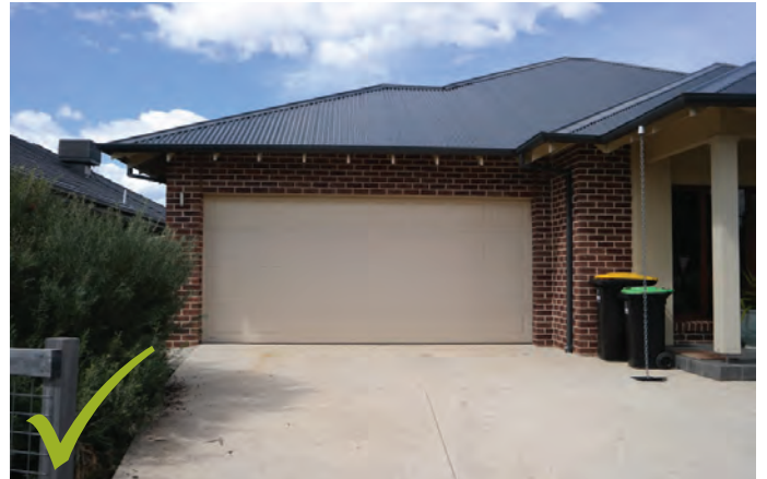
Example of compliant sectional panel lift door, and garage set back behind front facade.
