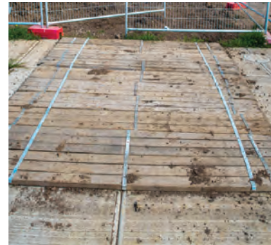
Example of wooden driveway crossover protection during construction of house.
