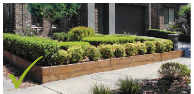
An attractive low retaining wall emphasised by planting.
